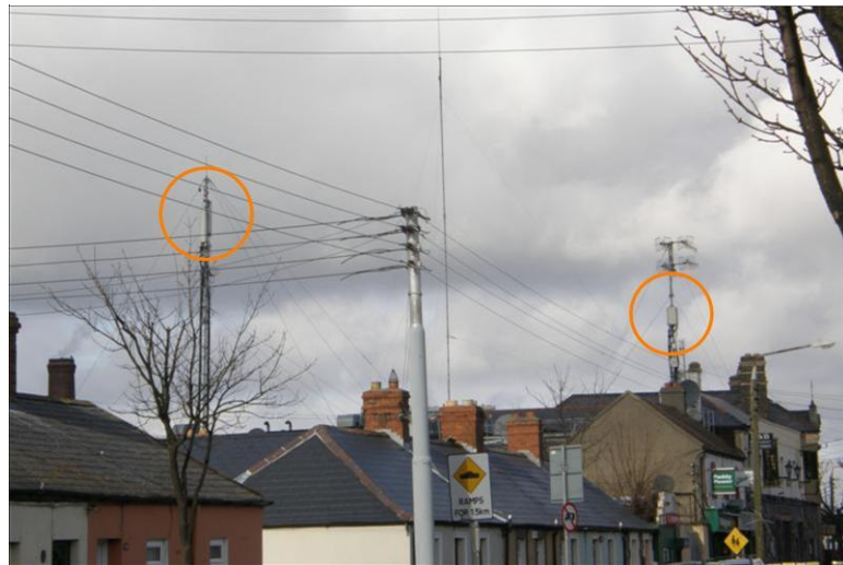
Transmitter Site Photo
